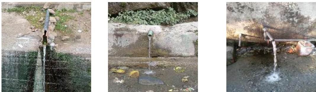
Fig. 2.8 Springs with piped outlet
